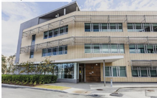
Building 8 – Dublin – Irlande
